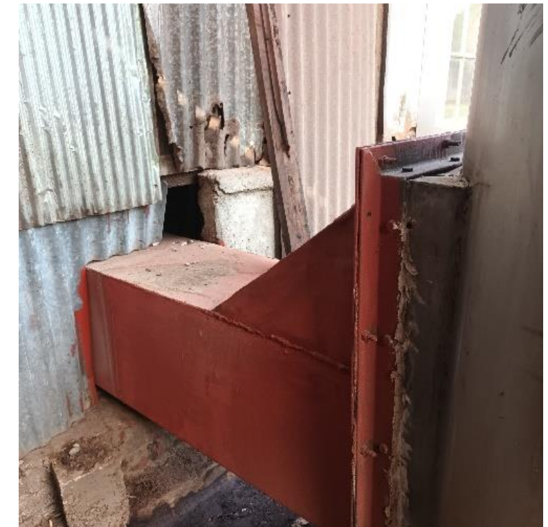
ID fan and flue gas line repair
