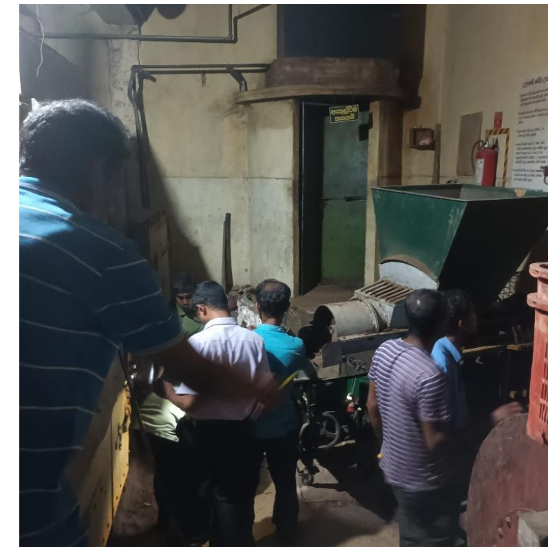
Retrofitting the unit to Air heater
