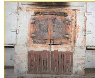
Ash pit door Properly placed
